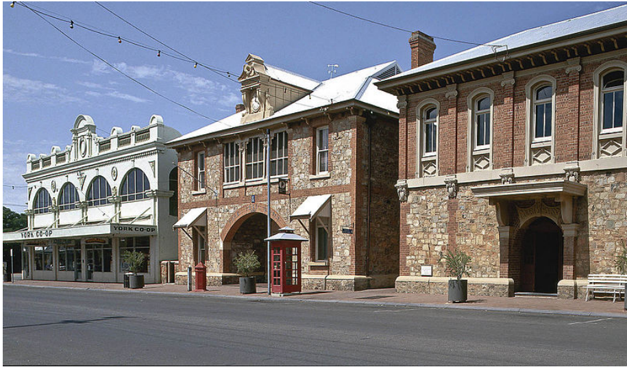
Figure 1: The Co-op, Post Office, and Courthouse on Stirling Terrace in York, Western Australia.
